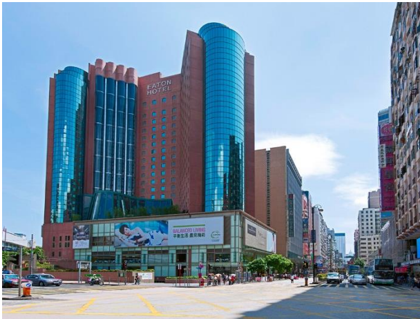
Eaton Hotel Chiller Upgrade Gold Award Hong Kong Awards for Environmental Excellence 2013
