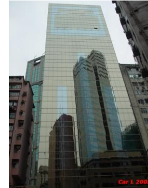
Typical Grade C office
