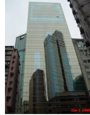
Typical Grade C office
