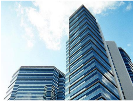
Typical Grade A office
