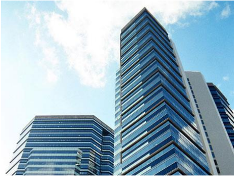
Typical Grade A office
